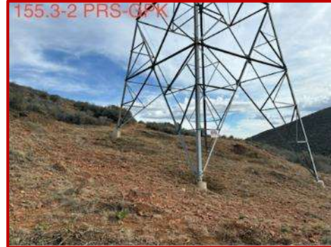
Figure 31 - WAPA Vegetation Clearance at Tower Base - Typical
